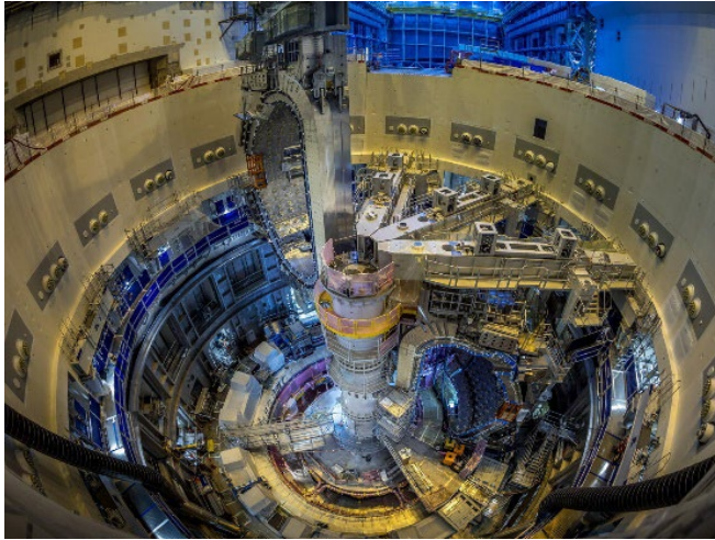
ITER Vacuum Vessel sector #8 is being lowered into the tokamak pit Source: ITER Organization
