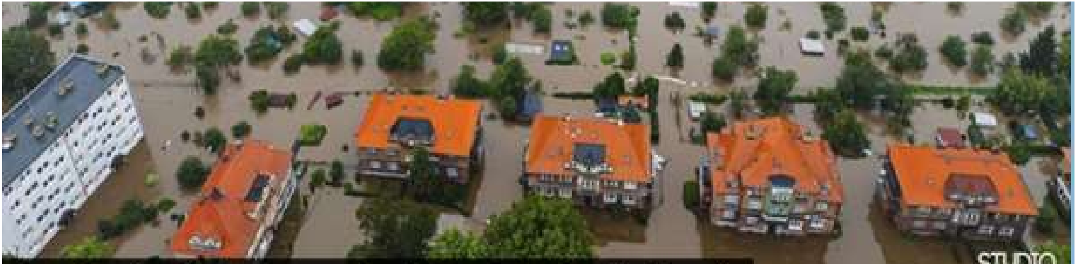
Poland - Flood September 2024 Source: State Water Management Polish Waters, "Report on the flood in 2024"
