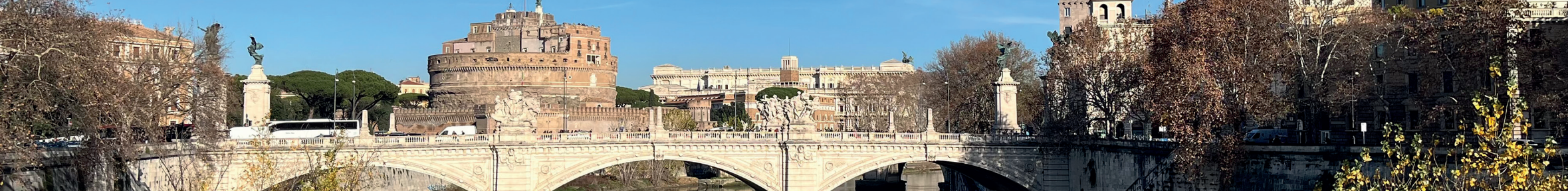
Ponte Vittorio Emanuele II, Rom © Florian Ambach.
