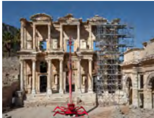
Start of conservation work on the Celsus Library in Ephesos (© OeAW-OeAI/N. Gail).
